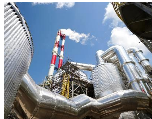
Sulfuric Acid Plant
