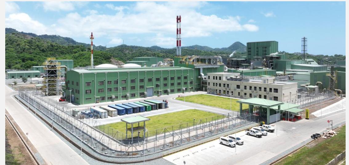
Smelter and PMR complex
