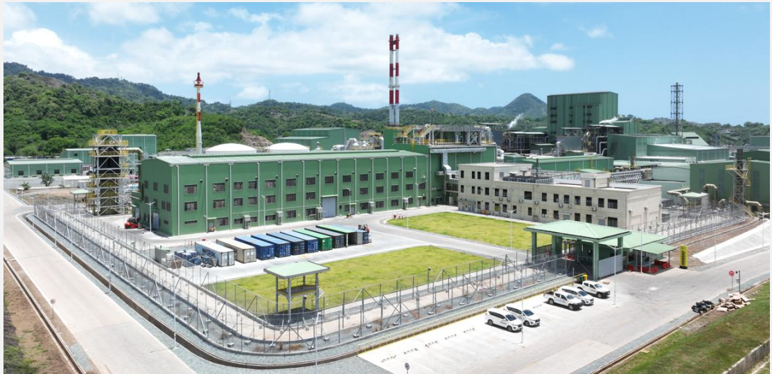
Smelter and PMR complex
