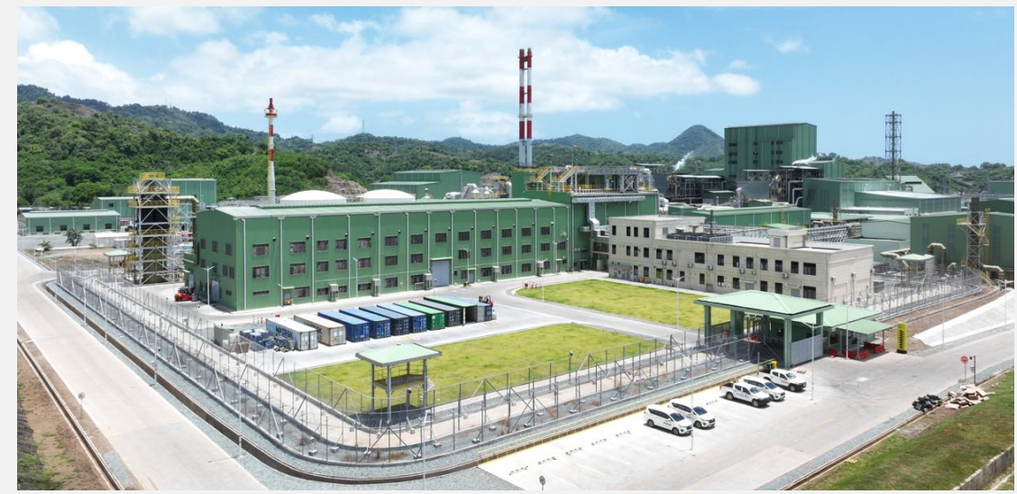
Smelter and PMR complex
