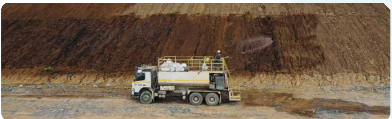
▲ Arranging and reshaping the piles using heavy machines.
