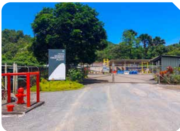
^ Sewage Treatment plant at our townsite.
