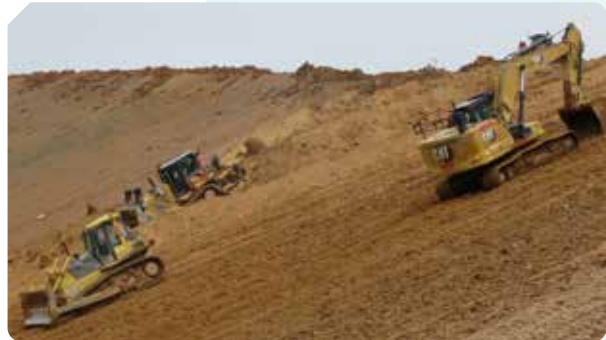
^ Soil placement (top) and soil compaction (bottom) using heavy machine.
