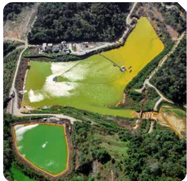
^ Holding pond for Acid Rock Drainage.
