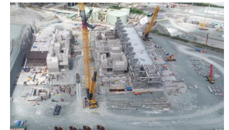
SAG and Ball Mill Foundations
