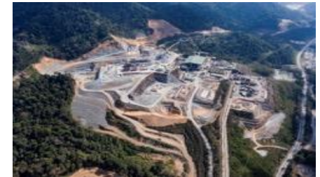
Processing Plant Area
